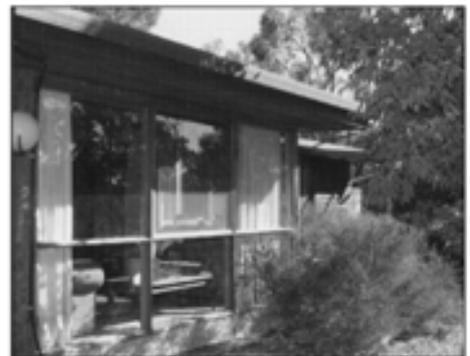
*Hazardous vegetation in close proximity to a building may increase the possibility of ignition through direct flame contact or radiant heat*
