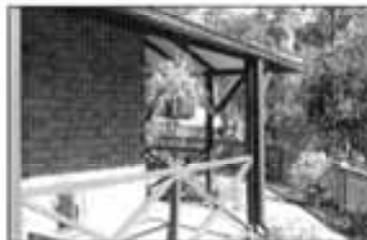
An unpainted wooden lattice may ignite more easily than a treated one.
