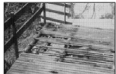
*Dry, untreated timber decking will ignite easily.*
